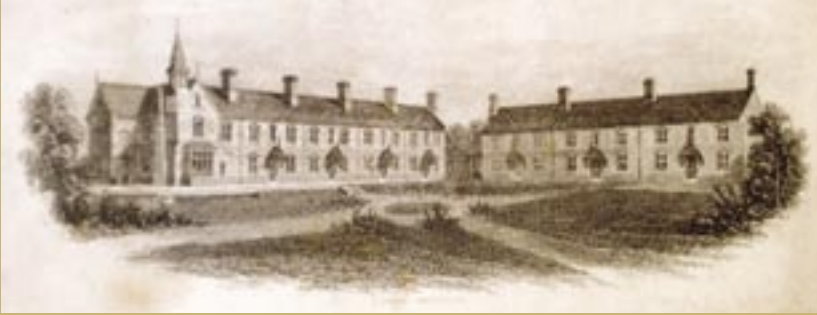
First phase of building, Southampton Road
